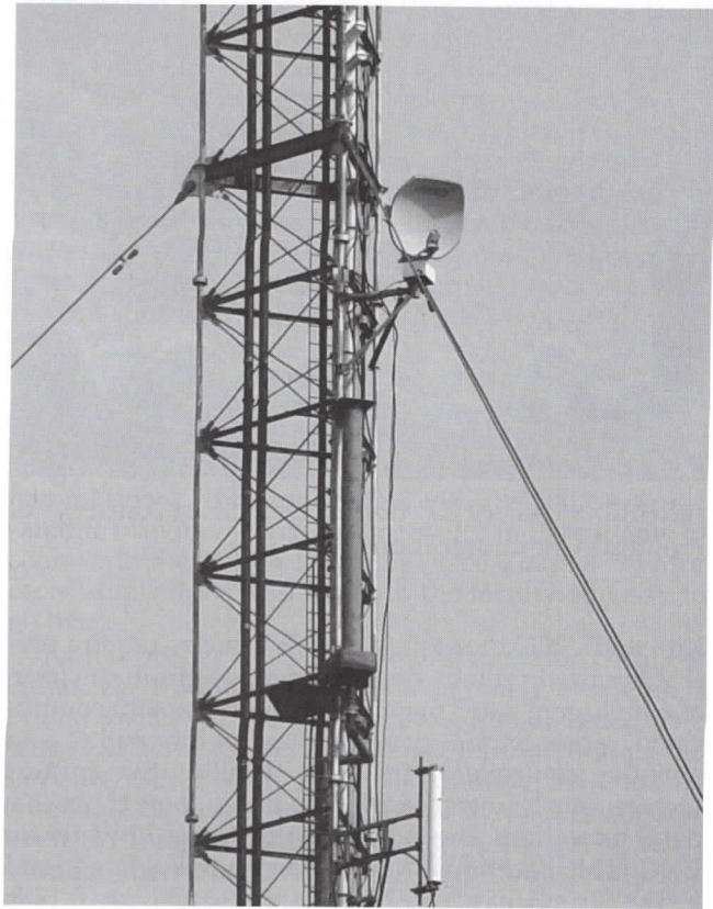
FIGURE 5.17-6 ENG remote-controlled receive antenna on tower.
