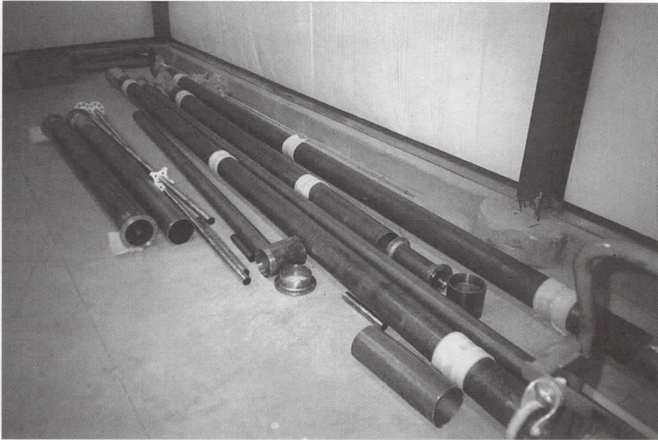
Figure 13.24 Disassembled rigid coax. Smaller-diameter copper is center conductor with dielectric spacers installed.
