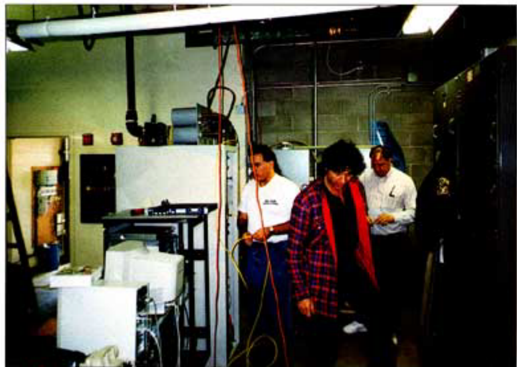
James Mueller, Chuck Pracna and David Lingenfelter install the transmitter and support equipment. Because the station did not have a digital STL, the ATSC encoder, multiplexer and SDI video source were installed at the transmitter site.
